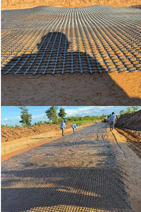
Gambar 5. Pemasangan geogrid MacGridTM EG S & EB
