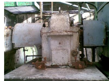
Gambar 1. Cover coupling motor to gearbox dan gearbox to pump
