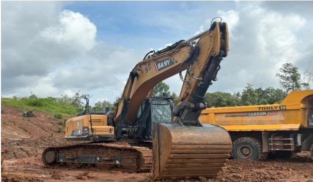
Gambar 8. Excavator Sany SY550HD
