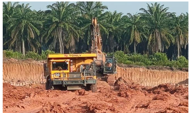
Gambar 3. Kegiatan Pengupasan Tanah Pucuk ( top soil )
