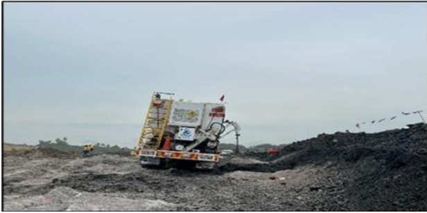
Figure 5. Filling blast holes with MMU
